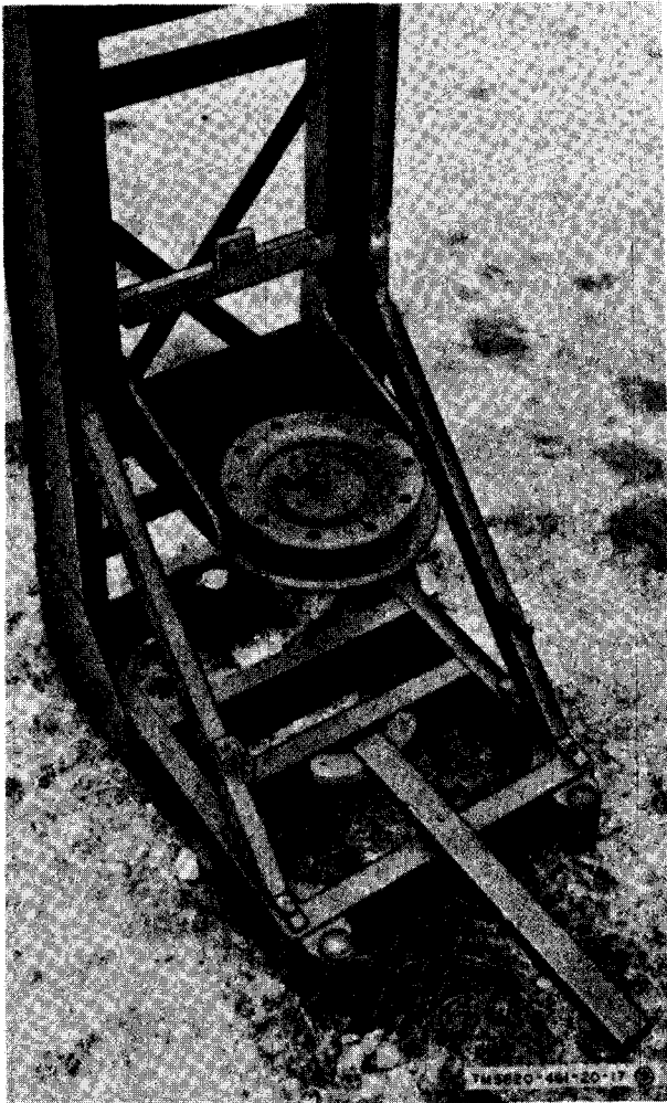
Figure 2-17Ⓣ. Erection of launcher (part 9 of 9)
