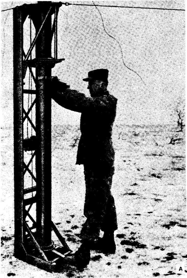
Figure 2-19②. Raising mast (part 2 of 4).
