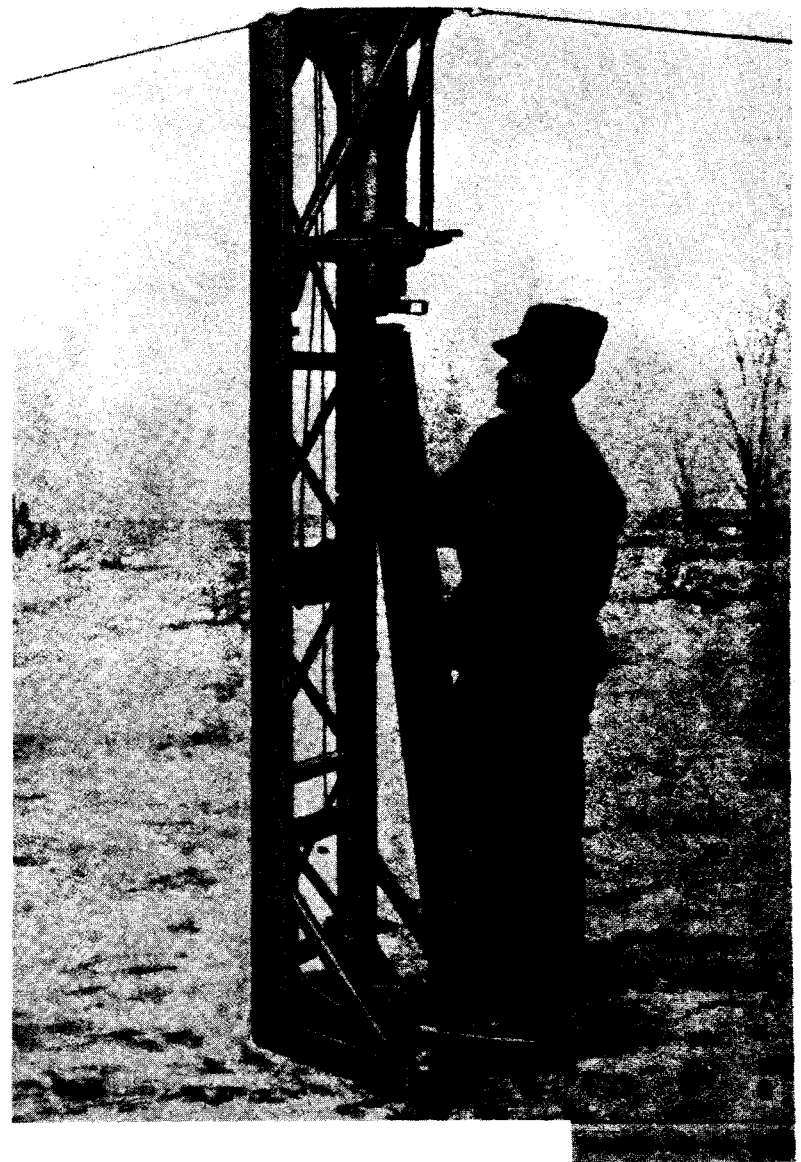
Figure 2-19①. Raising mast (part 1 of 4).
