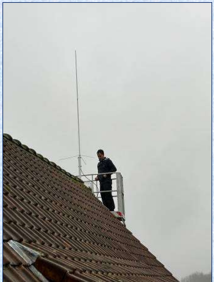
ON4PQ installed 144/430 MHz repeater antenna
